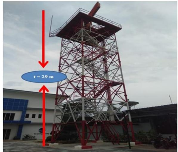
**Gambar 2.2 Antena RADAR MSSR MODE S**
